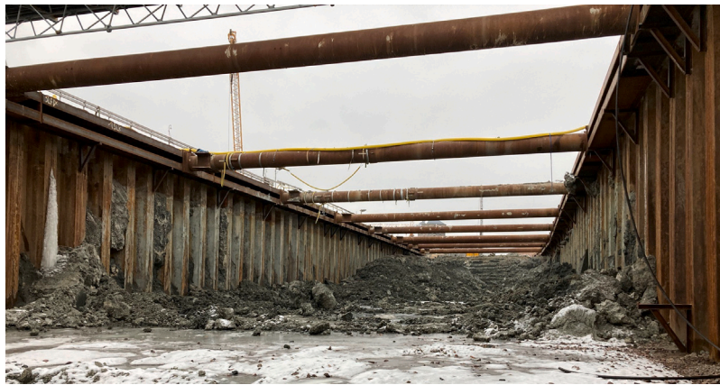
Fig. 11. The final excavation level of West Link excavation at KM:456+850 (Bozkurt, Sinem. West Link Project, Gothenburg. 16 Feb. 2021. Author's personal collection).
