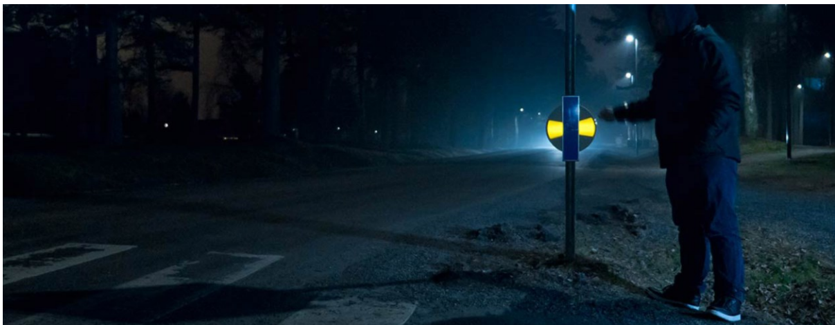
Figure 16: The Reflexsnurra device for visibility aiding at pedestrian crossings on unlit rural roads.
