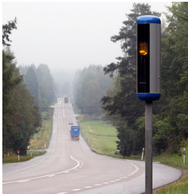
Figure 15: An automated traffic control camera (ATK: Automatisk TrafikKontroll). Image from Swedish Transport Administration (2023a).
