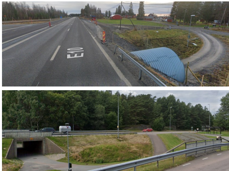
Figure 13: Examples of graded/grade separated crossings.
