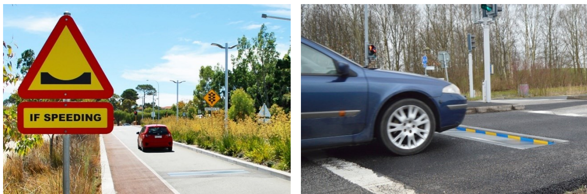
Figure 18: The Actibump system for dynamic urban speed control.
