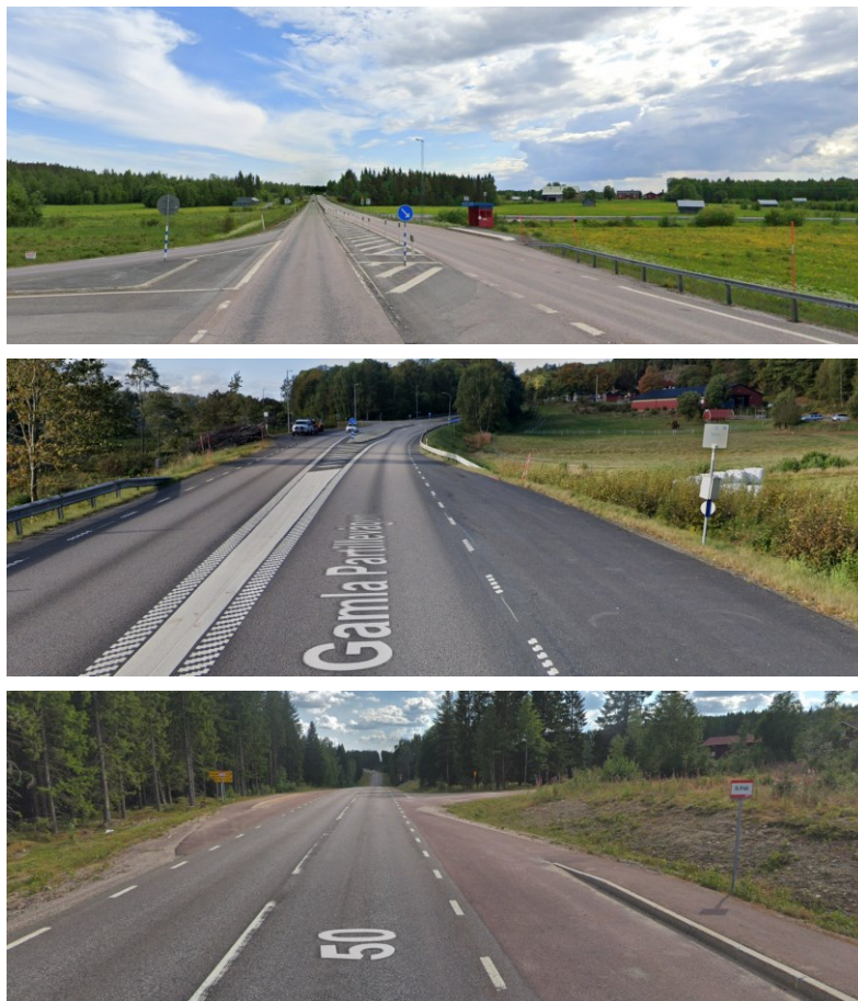
Figure 14: Examples of at-grade uncontrolled crossings.
