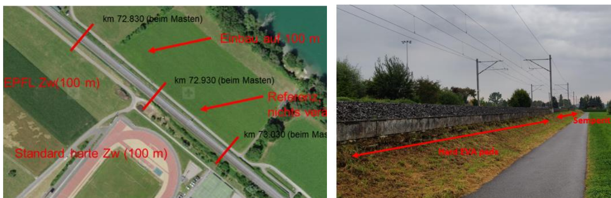
Figure 20: SBB test site: Left: an overview of the test site. Right: the track's surroundings.
