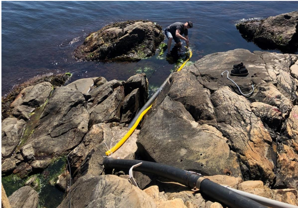
Figure 23. Establishing the hydrophone cable wear protection at the waters edge.
