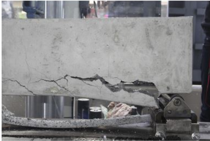
Figure 2.5: Concrete cover separation of FRP strengthened beam, permission from [22].
