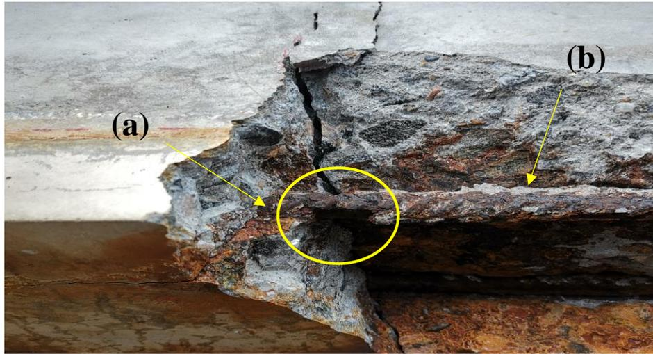
Figure 8: (a) Pitting corrosion. (b) General corrosion.
