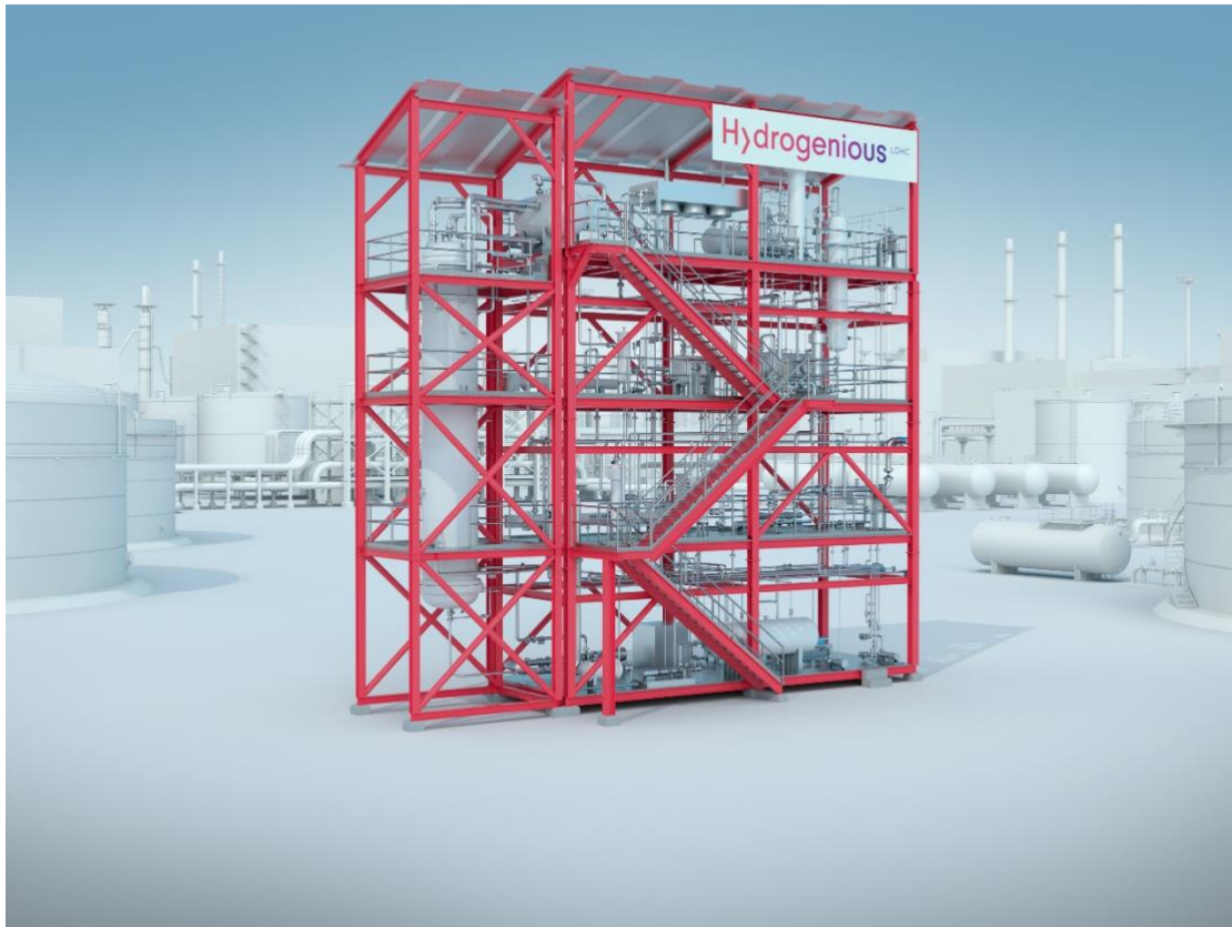
Figure 6. The LOHC storage plant developed by Hydrogenious LOHC Maritime (Figure from Hydrogenious LOHC Maritime, 2023).
