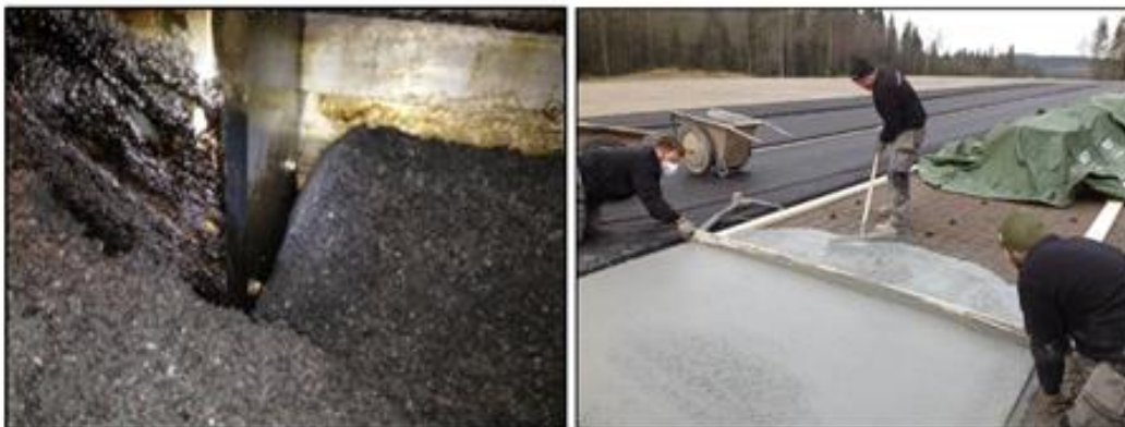
Figure 3.10. Rubber asphalt mixture (left), rubber concrete casting (right) [140] (License acquired through Copyright Clearance Center).
