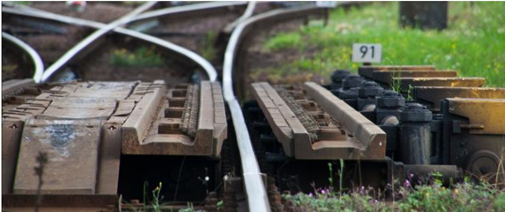
Figure 3: Ramp retarder in München-Nord [Source: jrschmidt-photos.de]
