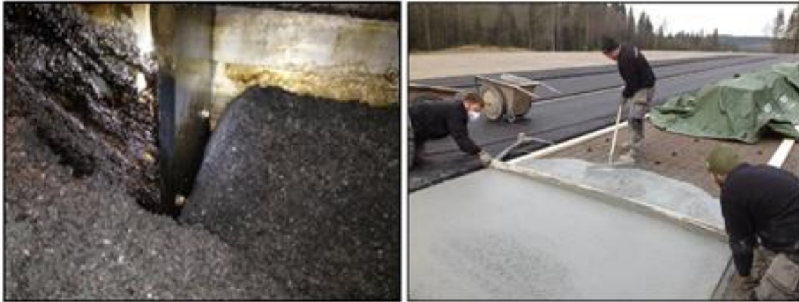
Figure 1.2. Rubber asphalt mixture (left), rubber concrete casting (right) [13] (Licence acquired through Copyright Clearance Center).
