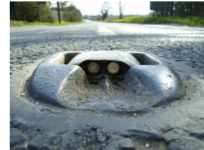
Figure 3. Cat's eye pavement marker.
