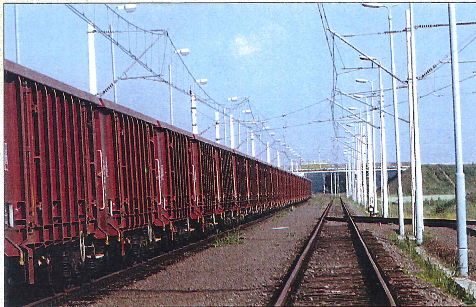
A heavy test train for testing permanent way and substructure of the track composed of tested wagons (if necessary).
