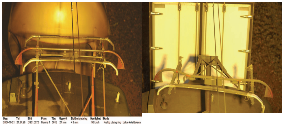
Picture 4.1 shows two examples of damaged pantographs (pictures provided by KIKA system).
