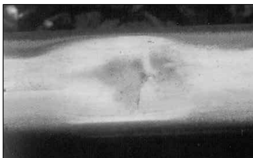
Figure 13: Squats in rails [Courtesy – V. Reddy, QUT, Australia]
