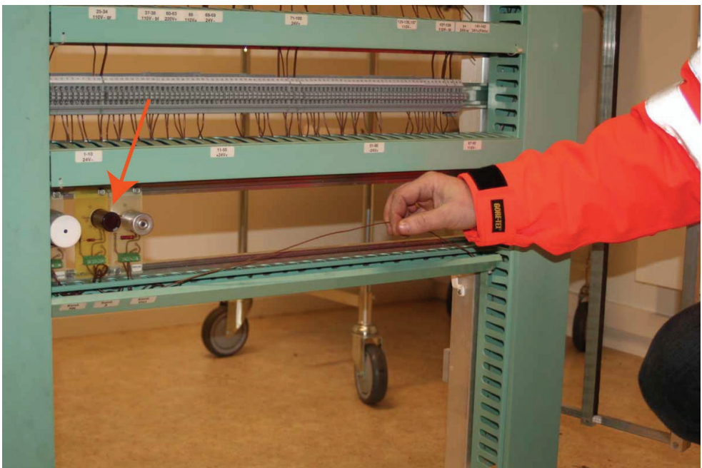
Figure 13 The placement of the RC circuit in the rack (the middle RC circuit in the square indicated by the arrow) and the wire from RC circuits that have the same size both on the negative bound and on the voltage side. The area of the solid wire is 0.75\ \text{mm}^2 .
