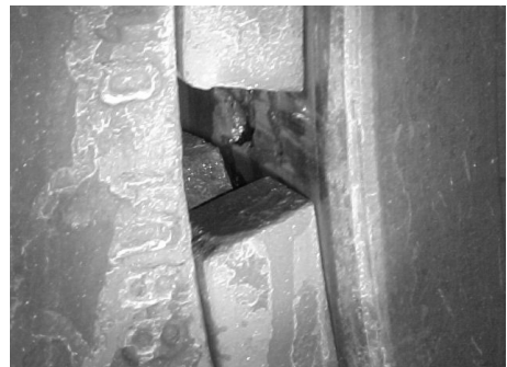
Figure 4. Damage identified between the brake pads (wheel seen to the right).
