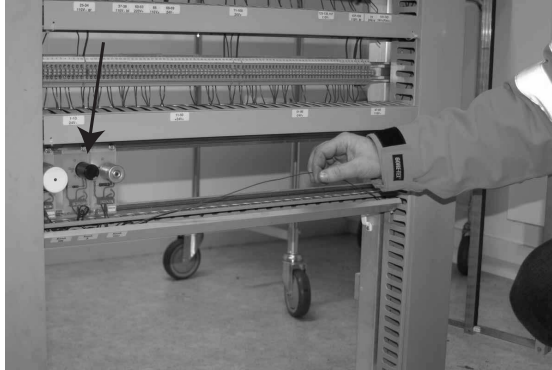
Figure 10: The placement of the RC circuit in the rack, by the arrow, and the wire from RC components that have the same size both on the negative bound and on the positive side. The area of the wire is 0.75 \text{ mm}^2 .
