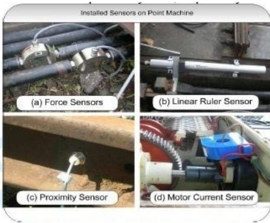
Figure 2. Installed Sensors on Turnout System
