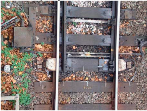
Figure 5: Electric Motor in Switch [3]
