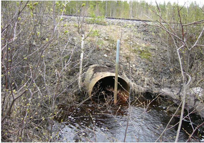
Figure 9: A culvert under the track
