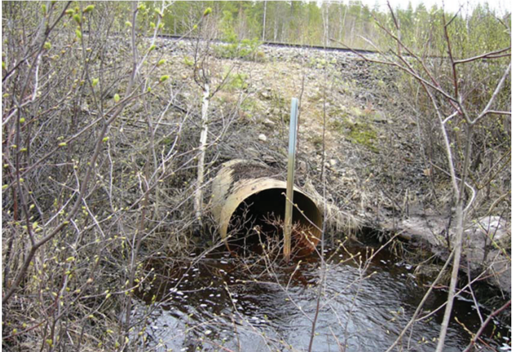
Figure 6.8 A culvert under the track
