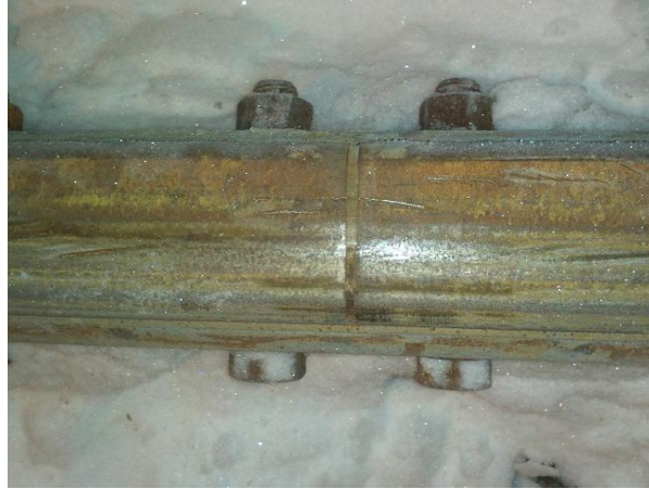
Figure 5. Insulated rail joint.
