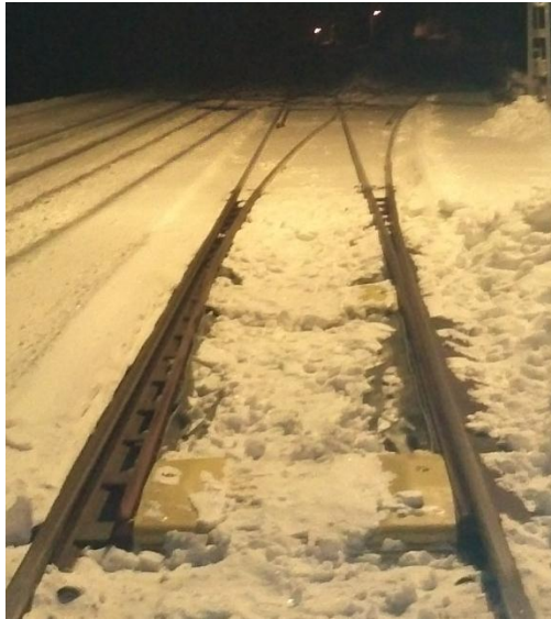
Figure 3. Switch on the track.
