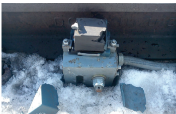
Figure 8: Failed sensor belonging to the wheel profile monitoring system (photo by Dan Larsson).
