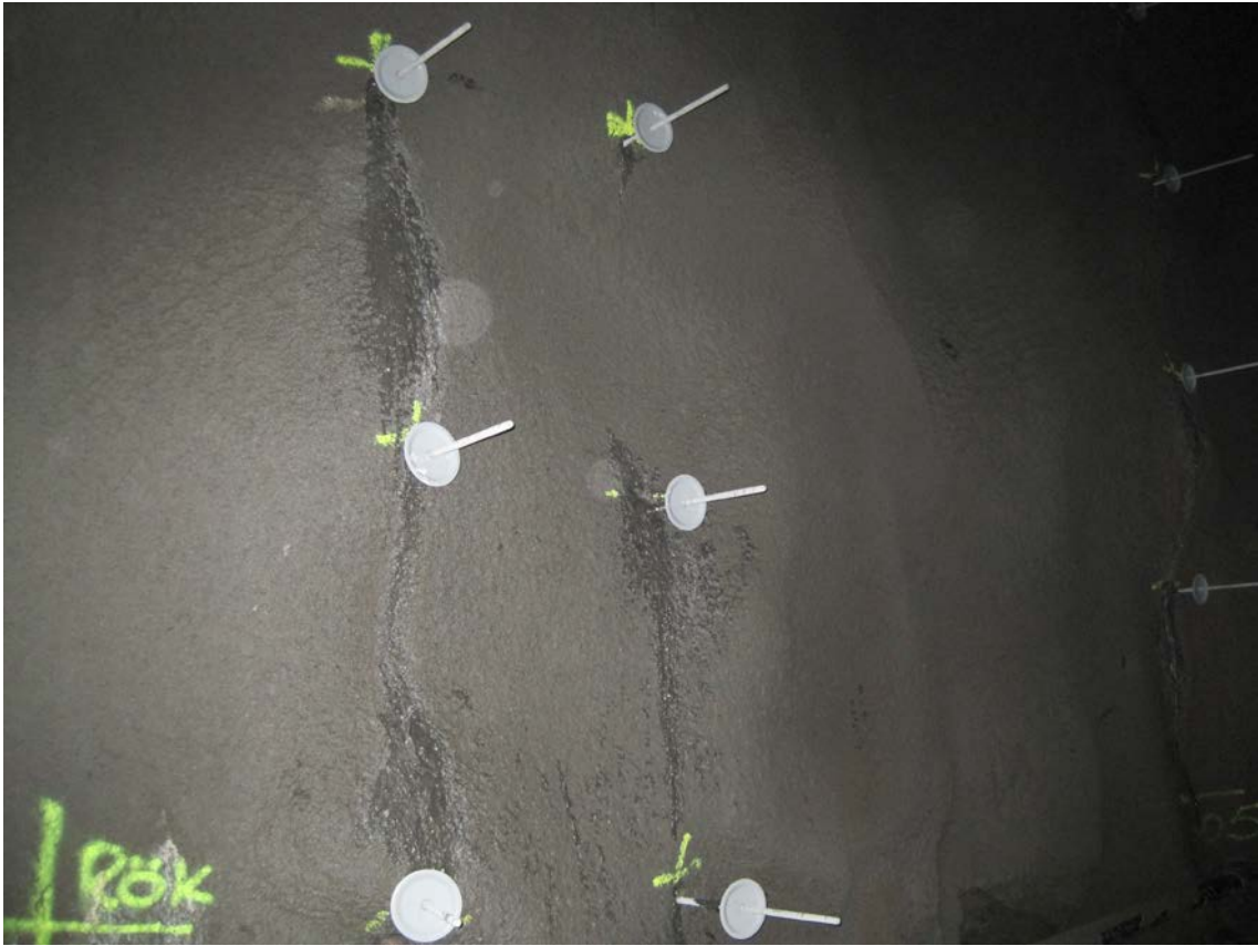
Figure 8 Mounted threaded rods ready for assembly of the standard drainage.
