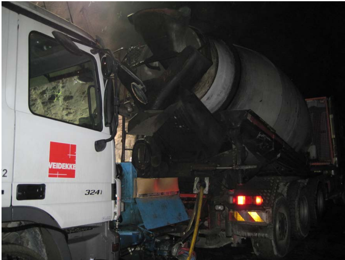
Figure 3 Filling of ordinary premixed shotcrete in the spraying robot.
