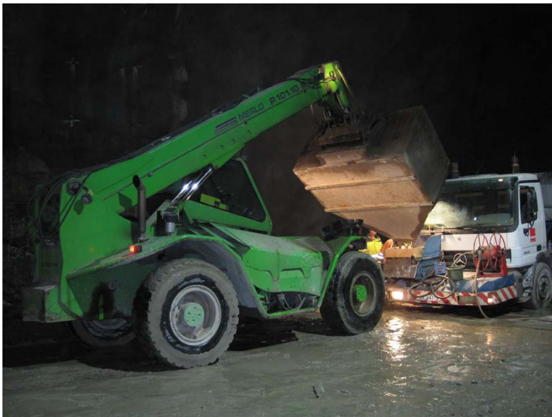
Figure 4 Filling of Solbruk T shotcrete in the spraying robot.
