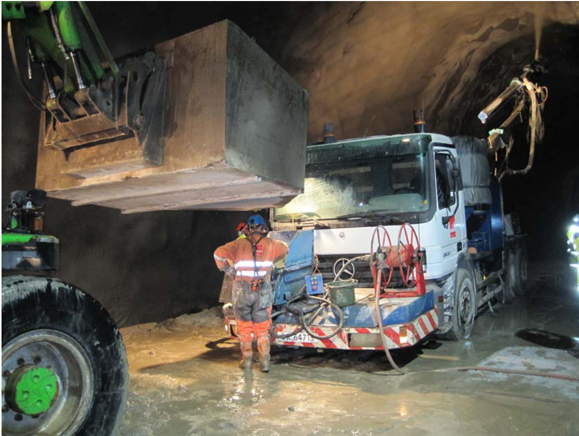
Figure 5 Shotcreting with Solbruk T shotcrete.
