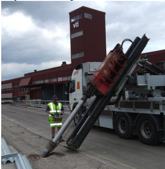
Punching of holes for an inclined barrier.
