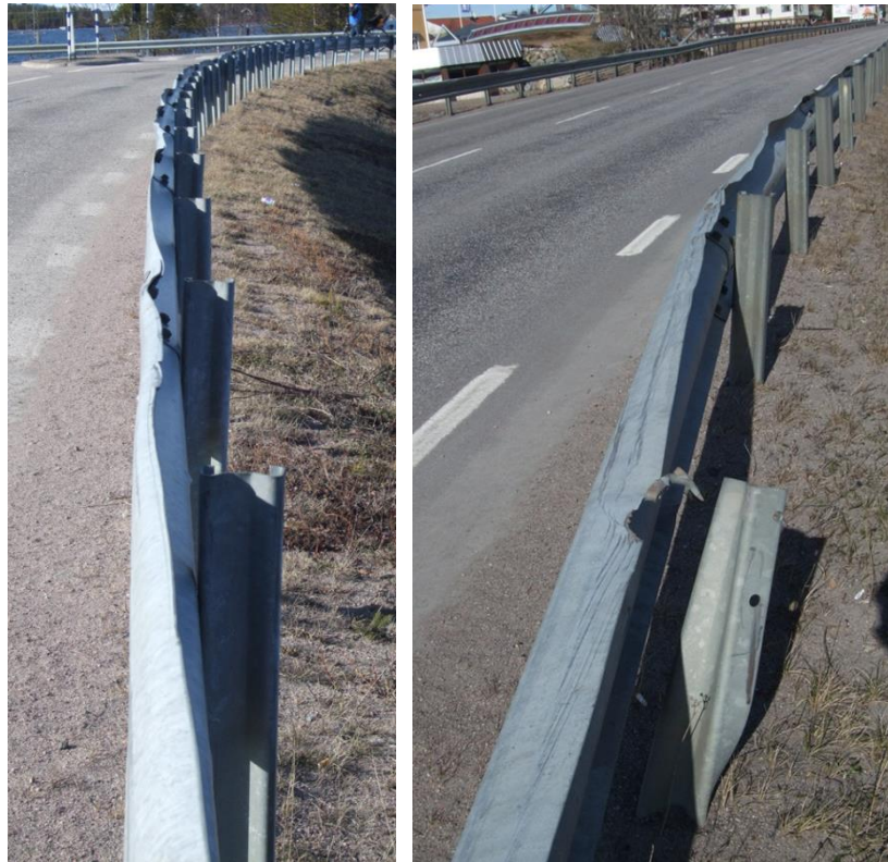
Examples. W-profiles deformed from snow removal.
