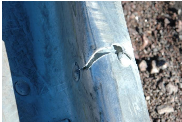
Barrier was too low and too angled, bolts did not shear off, resulting in a breach of barrier. Did see cracks and tear of the cross member.
