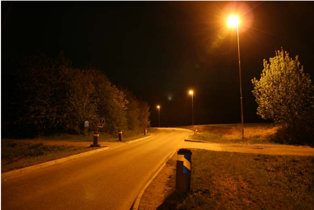
Figure 6 The pinkish-orange high pressure sodium lamps (HPS) is the most widely used lamp type in street lighting.
