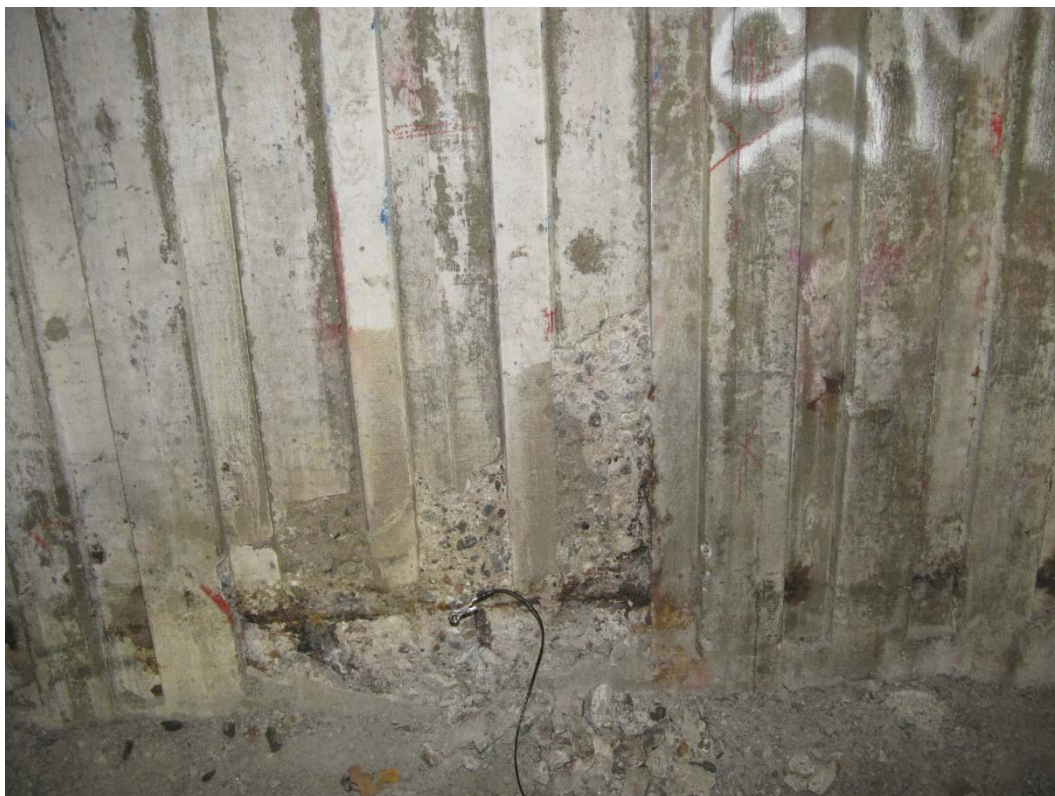
Figure 5.2.5 Black cable connection in the first measurement.
