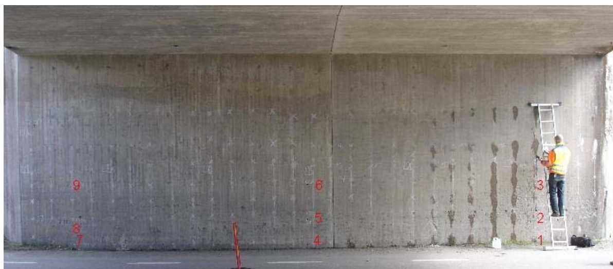
Figure 5.4.7 A view of the measurement area on the eastern front wall of Bridge 19-380-1 [Lind & Wikslund, 2010]
