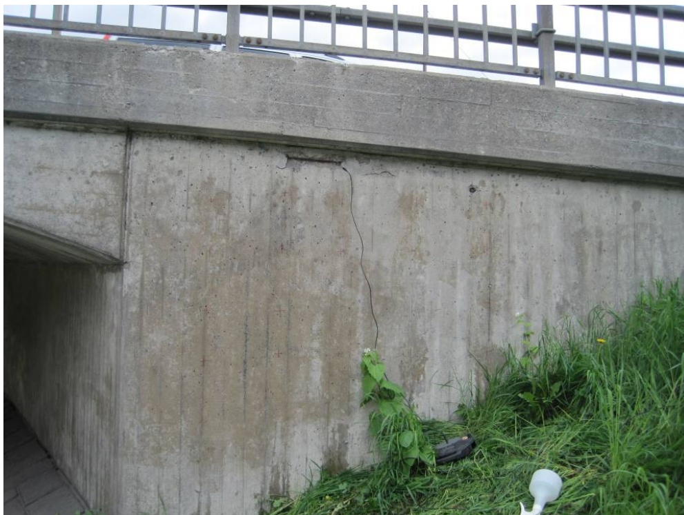
Figure 5.3.11 View of the measurement area on the wing wall of Bridge 7.
