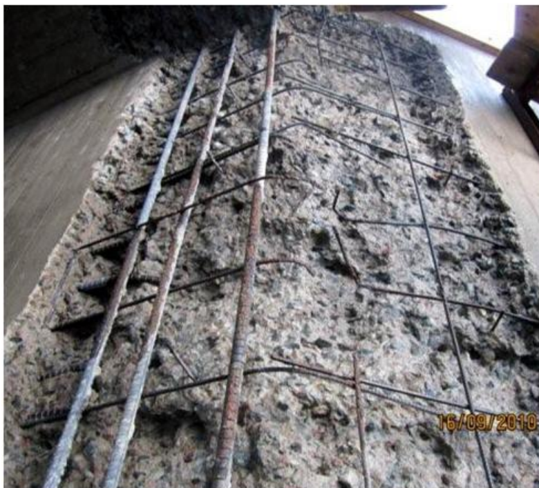
Figure 5.4.12 Reinforcement bars after removal of concrete at the southern opening of the eastern front wall of Bridge 19-380-1 [Lind & Wikslund, 2010]
