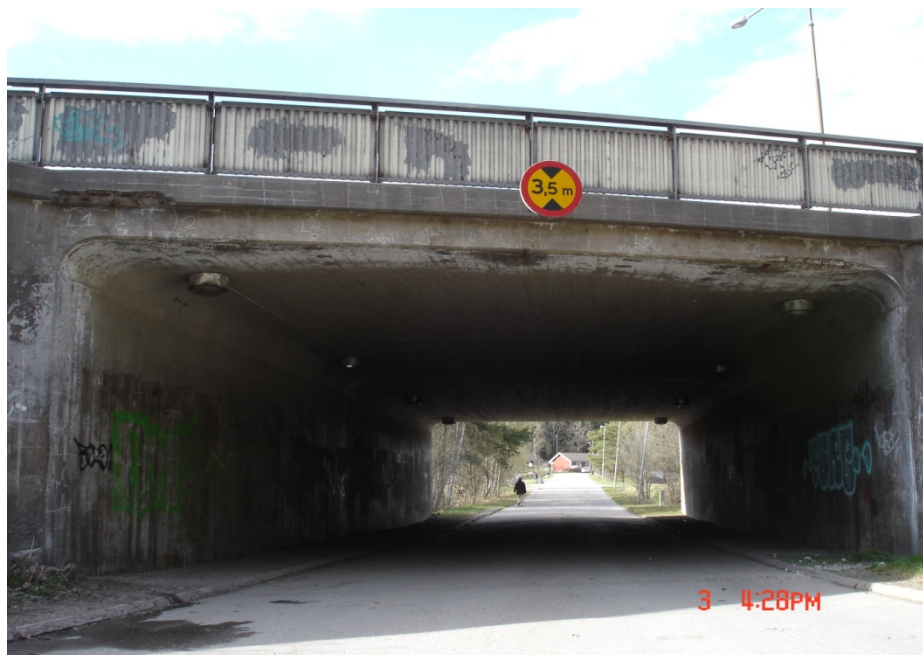
Figure 5.4.18 A view of Bridge 19-386-1 from the south side [Lind & Wikslund, 2010].
