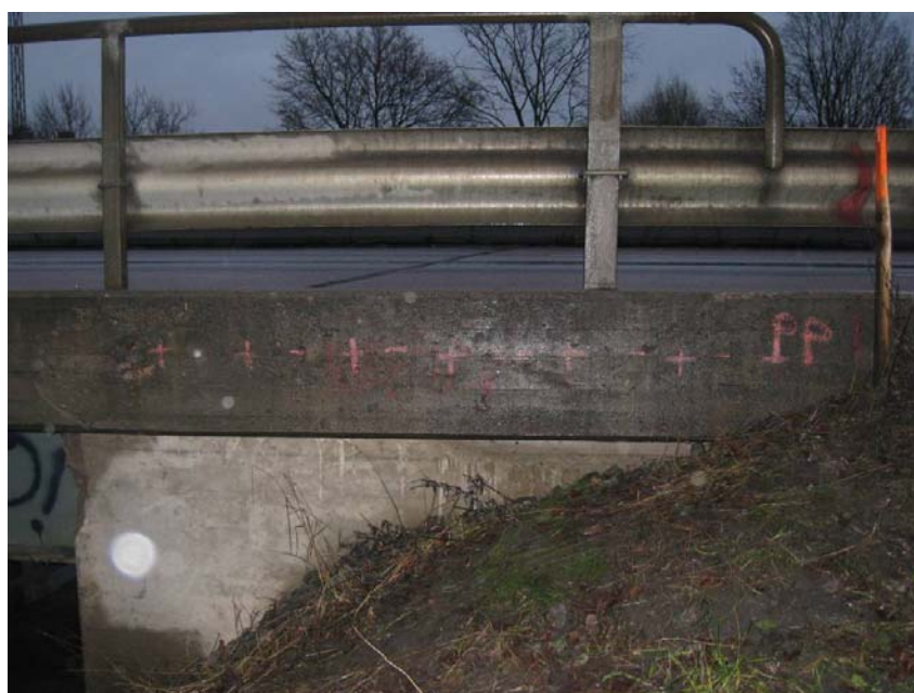
Figure 5.3.5 View of the measurement area on the edge beam of Bridge 5.
