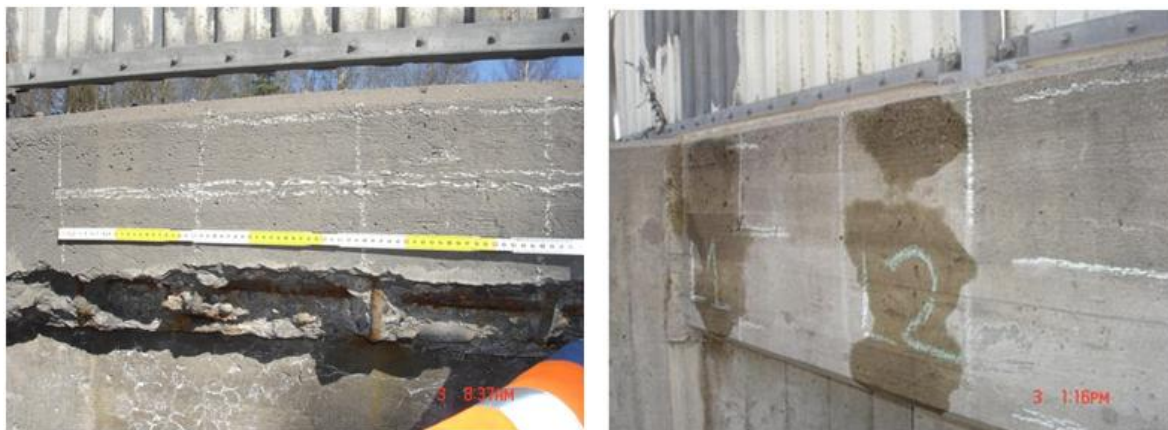
Figure 5.4.19 Measurement grids on the southern edge beam (left) and the northern edge beam (right) of Bridge 19-386-1 [Lind & Wikslund, 2010].
