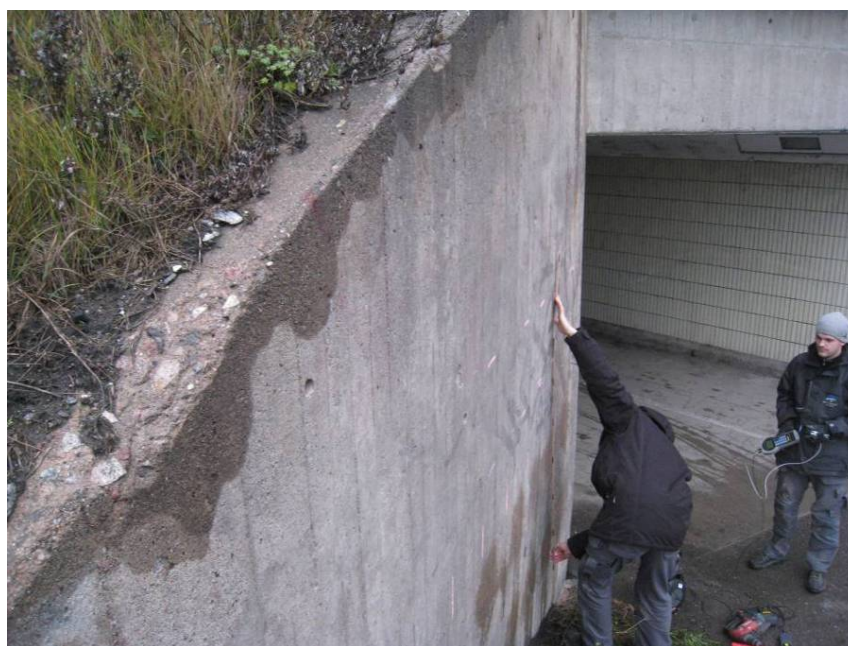
Figure 5.3.3 View of the measurement area on the wing wall of Bridge 3.
