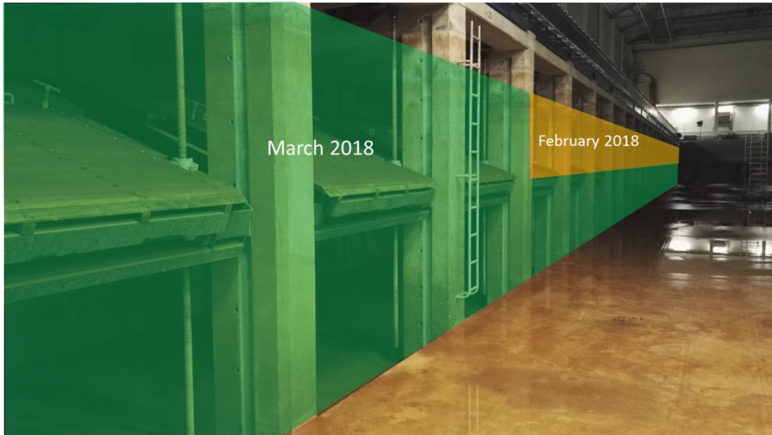
Figure 9: Two stages of covering the pillars
