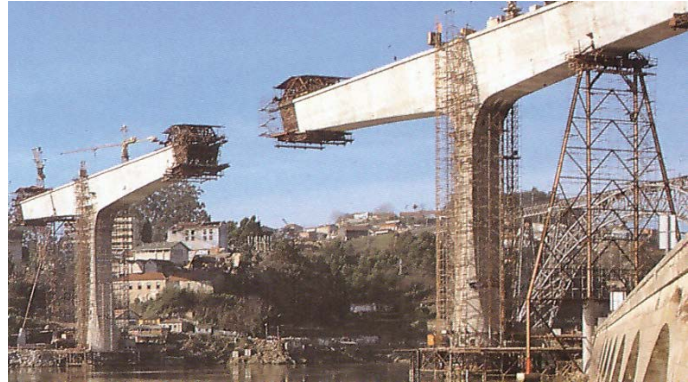
Figure 7.5 Photos from the new railway bridge in Porto shows preparation for extra external post-tensioning, (Nova ponte ferroviaria sobre o Rio Douro no Porto)
