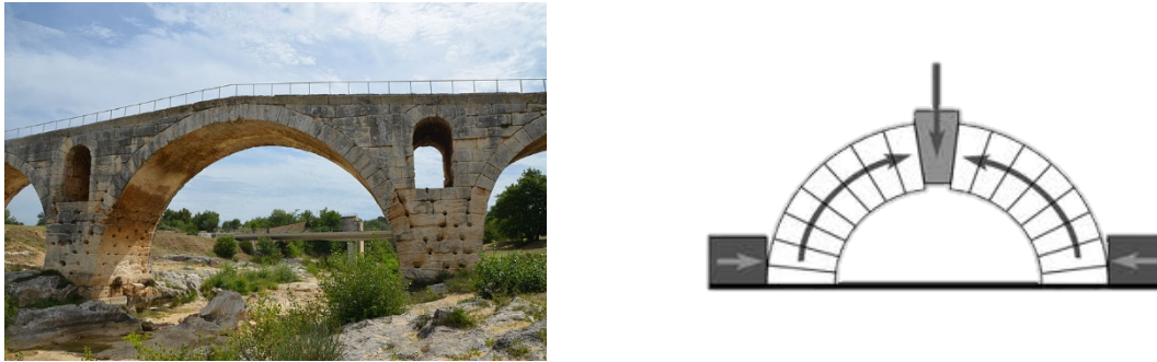
Figure 2.1. Load-bearing principle for an arch with mainly compressive stresses, www.wikimedia.org and Nilsson (2014).
