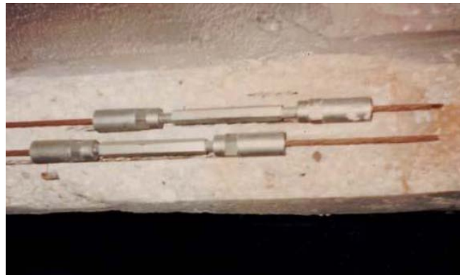
Figure 7.6 Strand splice, (Harris et. al., 2009)
