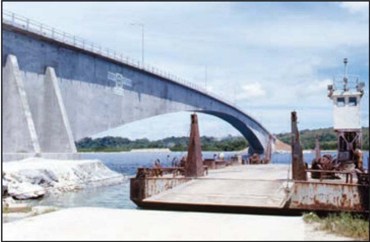
Figure 6.4 The 249 m span of the prestressed Koror bridge (and the ferry it replaced) before failure in 1996 due to creep and relaxation, Tang (2014).
