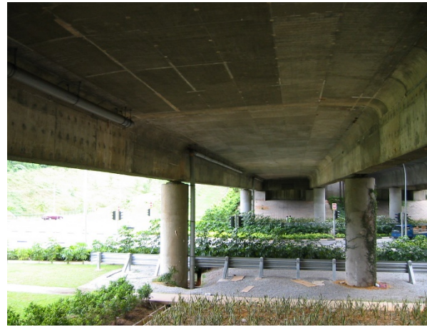
2 continuous main girders seen from below. Before external prestressing
