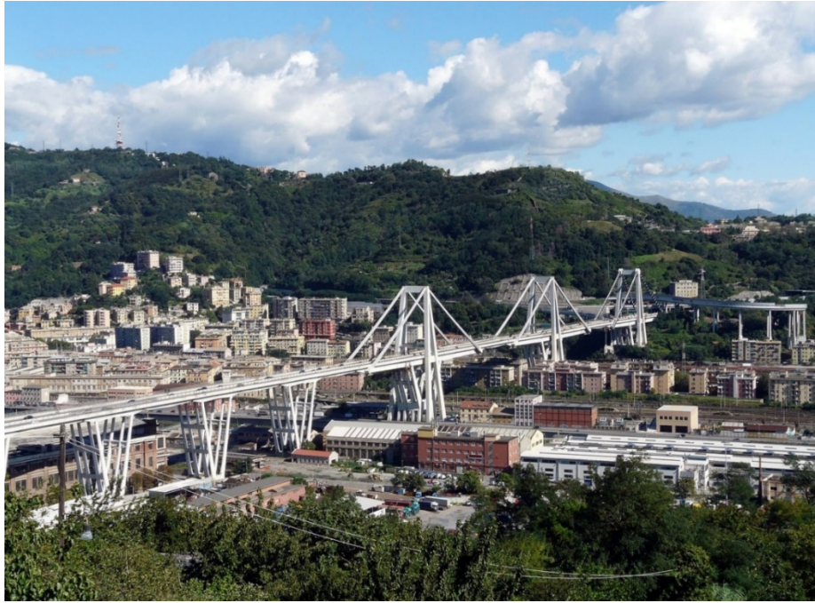
Figure 3.8. The Polcevera bridge in Genoa, Italy, from 1967, designed by Ricardo Morandi, partly collapsed on August 14, 2018. A cable stay broke in the tower to the left in the picture, probably due to corrosion and fatigue caused by cracks in the prestressed concrete supposed to protect it, see Figure 3.9. Photo by Davide Papalini, https://commons.wikimedia.org/w/index.php?curid=11542499
