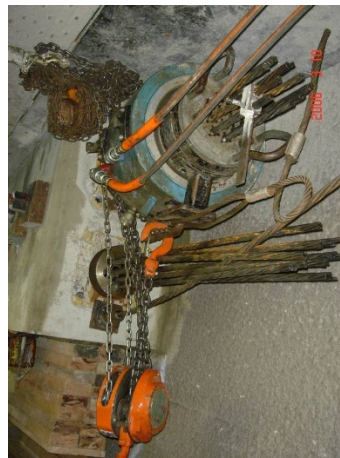
Prestressing of cable at top - "live end". "Dead end" for cable at bottom.
