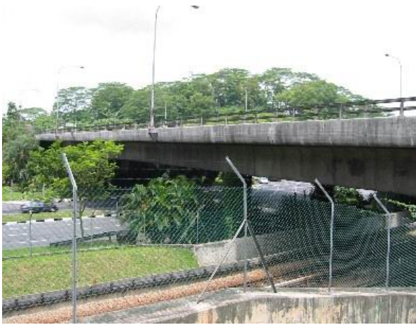
Woodland flyover. 3 span bridge with 2 main girders and bridge deck slab.
