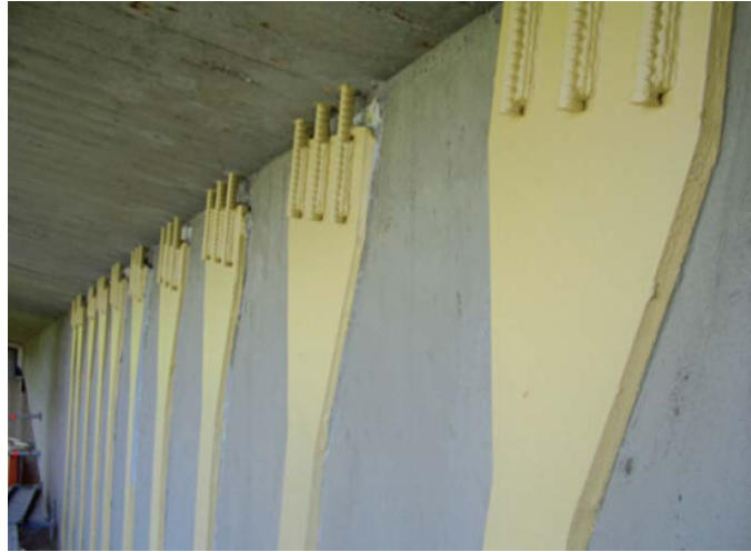
Figure 7.7 Shear strengthening of a concrete bridge in Germany (Rose and Kerkeni, 2010)
