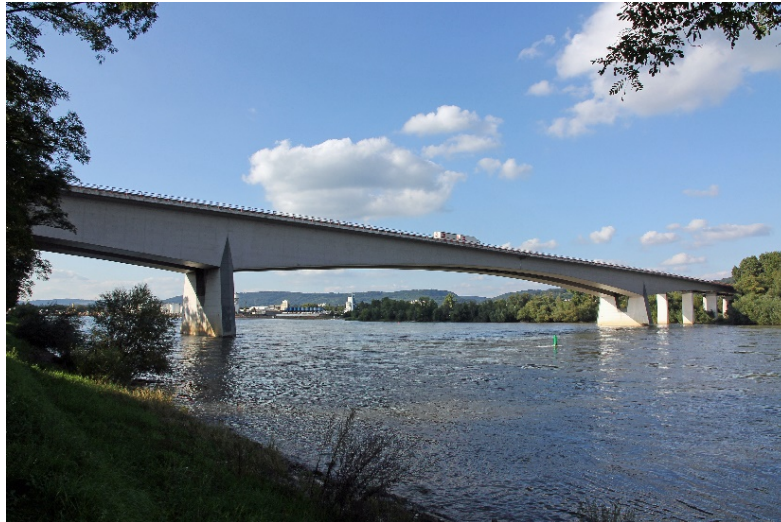
Figure 2.5. Free cantilevering bridge with a span of 202 m from 1962 by Ulrich Finsterwalder. Rhine near Bendorf and Koblenz Photo by Holger Weinandt 2014, Wikipedia.
