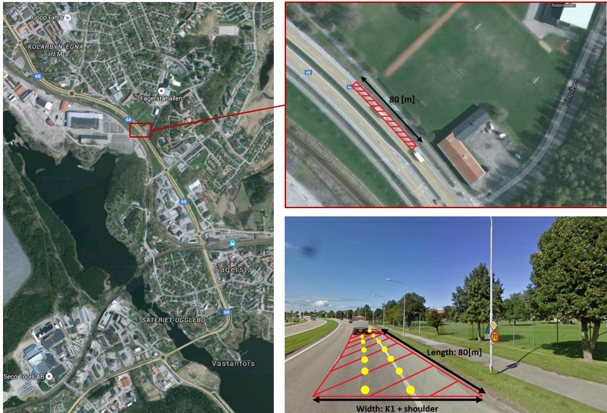
Figure C 1: The part of the test road, RV68 in Fagersta, where the magnetic markers have been mounted.
